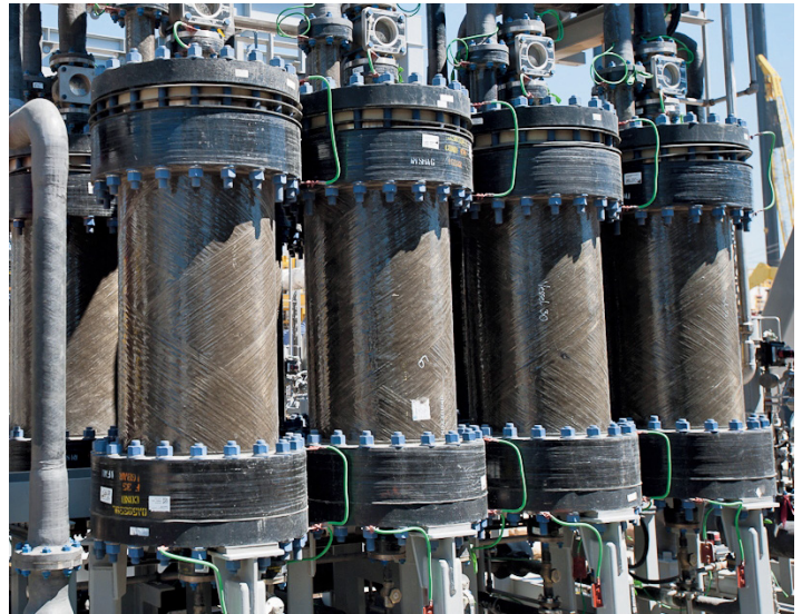
UF membrane housing vessels.
