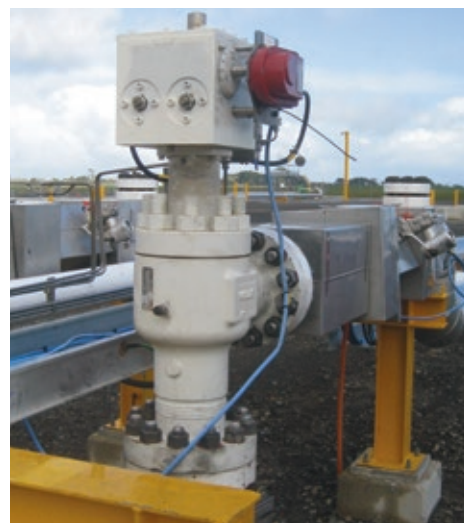
CC40 choke with hydraulic stepping actuation
