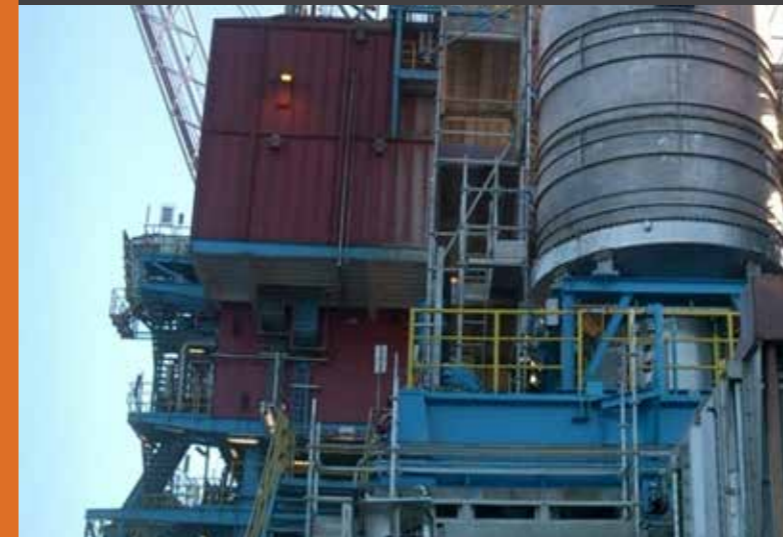
CiBAS: 49 tonne. Support structure: 4 tonne
