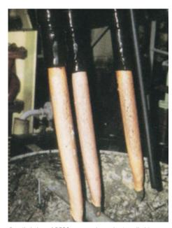
Detailed shot of BFCC system electrodes installed in a marine (strainer-type) system.
